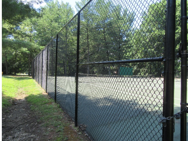
Tennis court fence
