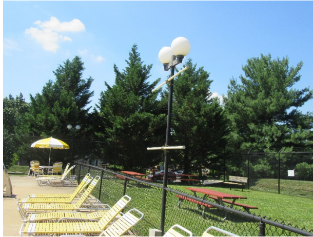
Light pole and fixtures
