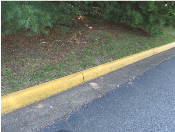
Concrete curb and gutter
