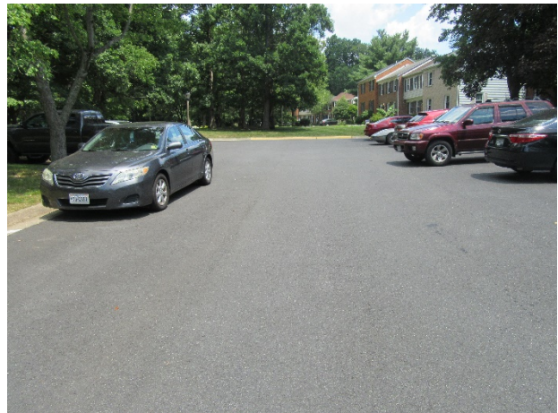
Asphalt pavement at Brainerd Court
