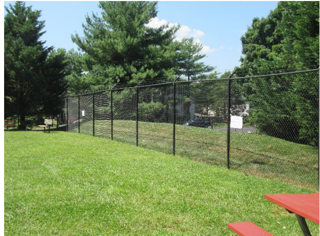
Chain link fence
