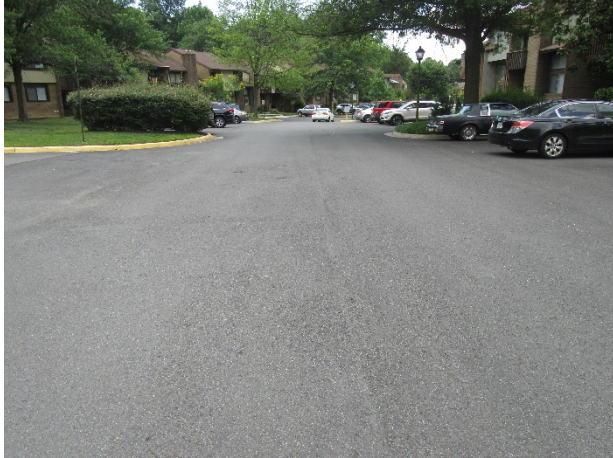
Asphalt pavement at Gwynedd Way
