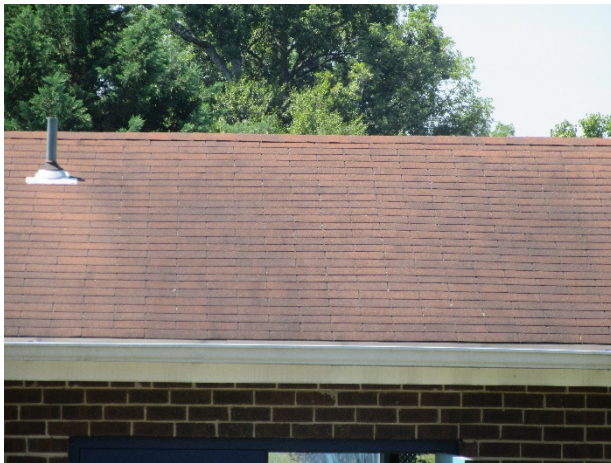
Asphalt shingle roof assembly
