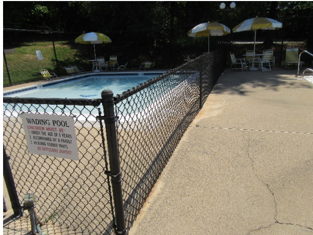
Chain link fence
