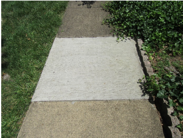
Concrete sidewalk partial replacements
